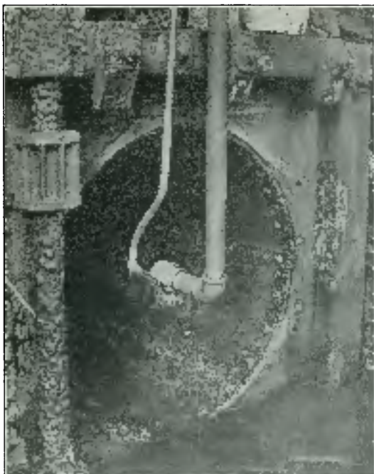
FIG. 2 HEAD GATE, MOUTH OF PENSTOCK AND 2-IN. QUICK-ACTING VALVE
